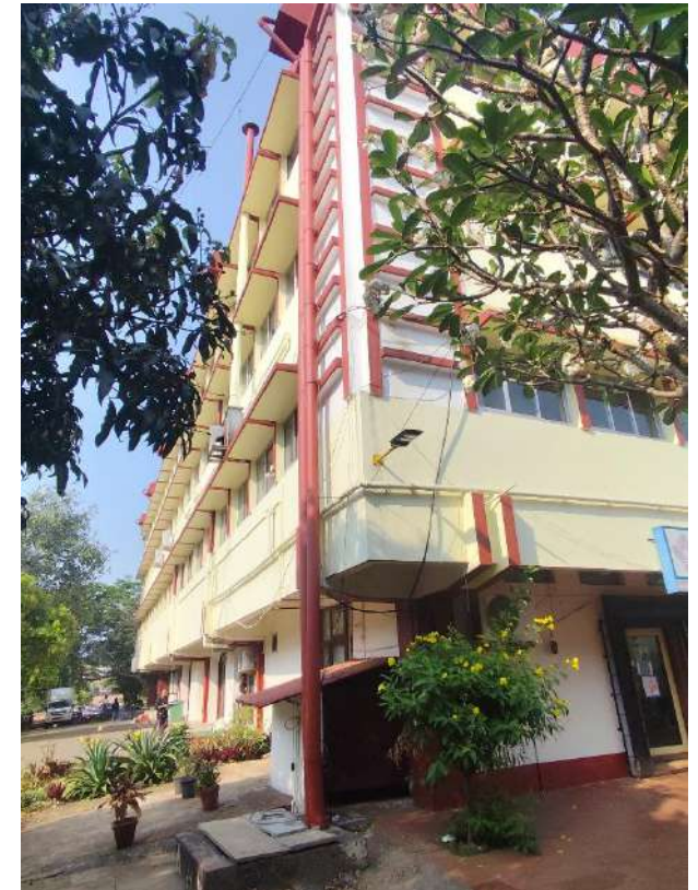
Downpipe for rainwater storage
