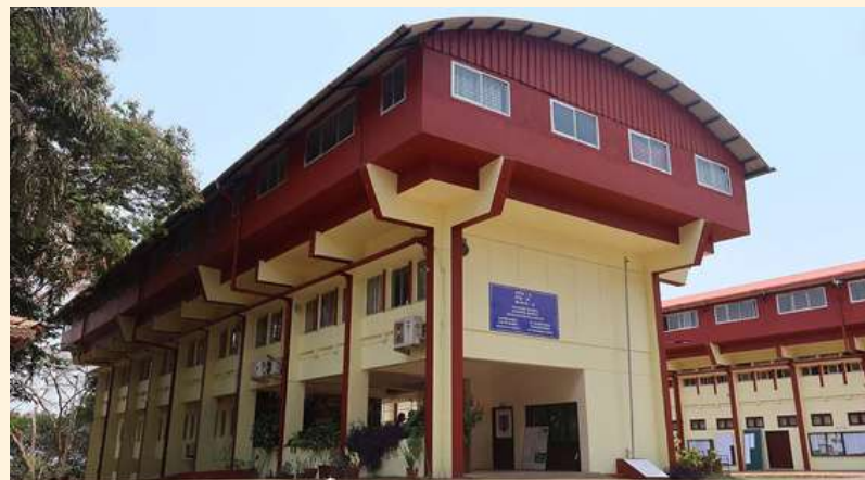
Administrative Block A
