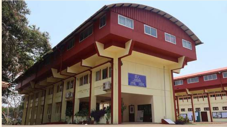
Administrative Block A
